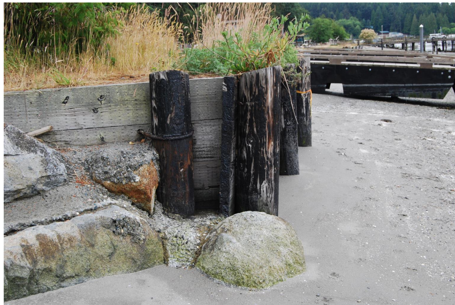
Creosoted bulkhead. Photo courtesy of the Northwest Straits Initiative.
