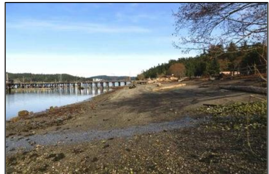
Figure 4. Photo of restored shoreline taken at on March 4, 2013. Bulkhead and fill removed and shoreline topography restored to enhance nearshore habitat for fish and other species.
