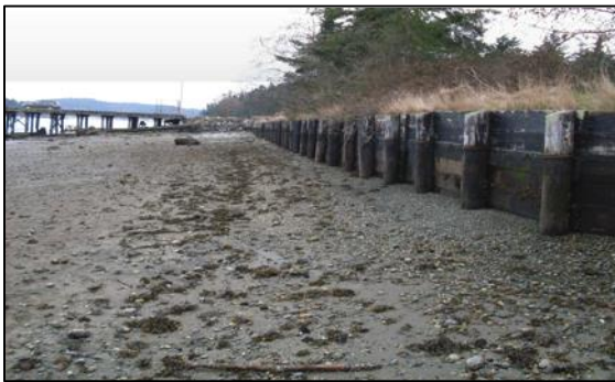
Figure 3. Photo looking northeast at modified shoreline, including bulkhead at the west end of the project area prior to restoration. Photo taken at established Photo Monitoring Station 1 on March 20, 2009.
